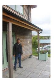
Above: The South-facing front of a three bedroomed house with plenty of glazing to capture the sun's heat. Inside it falls onto a black, melamine-covered concrete floor to absorb the heat.
